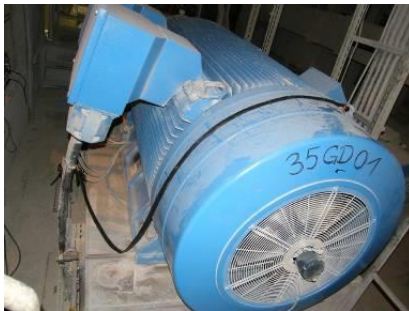
Paper plant Converter A Power: 1900 kW Motor A SH: 560 mm
