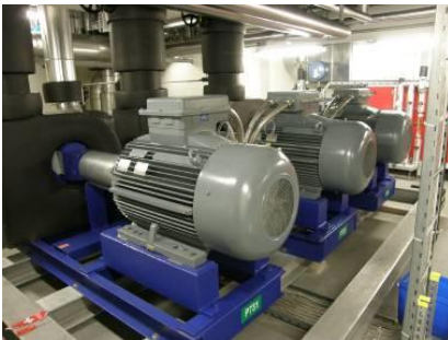
Pump Converter B Power: 160 kW Motor B SH: 315 mm
